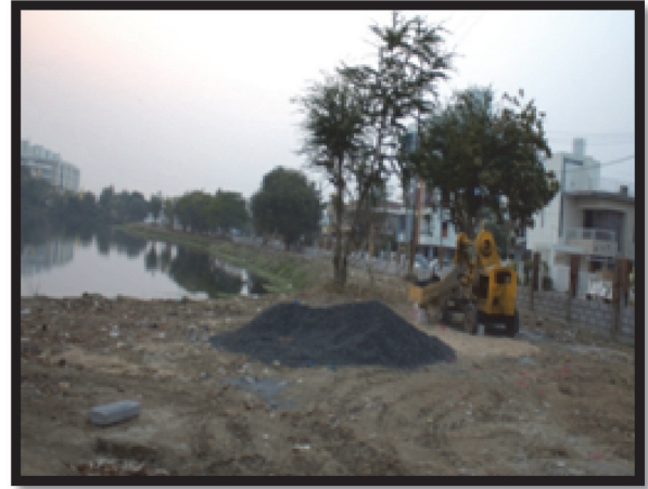
Construction around Urban Pond ( Harni Pond)
